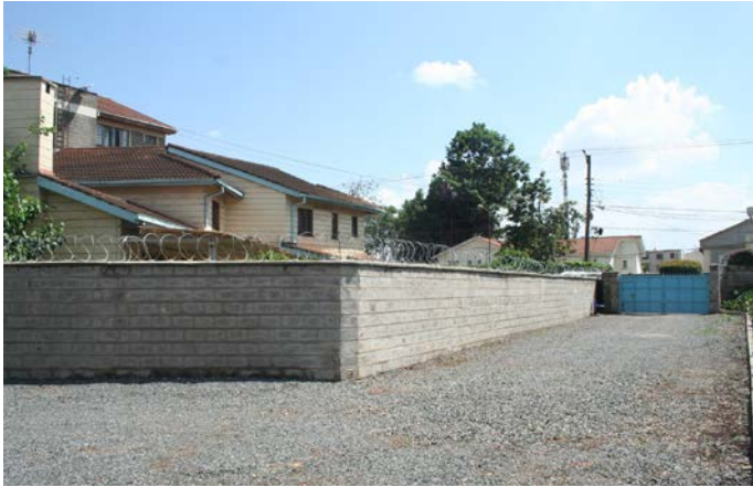
Perimeter-wall enhancement at the General Adviser's residence
